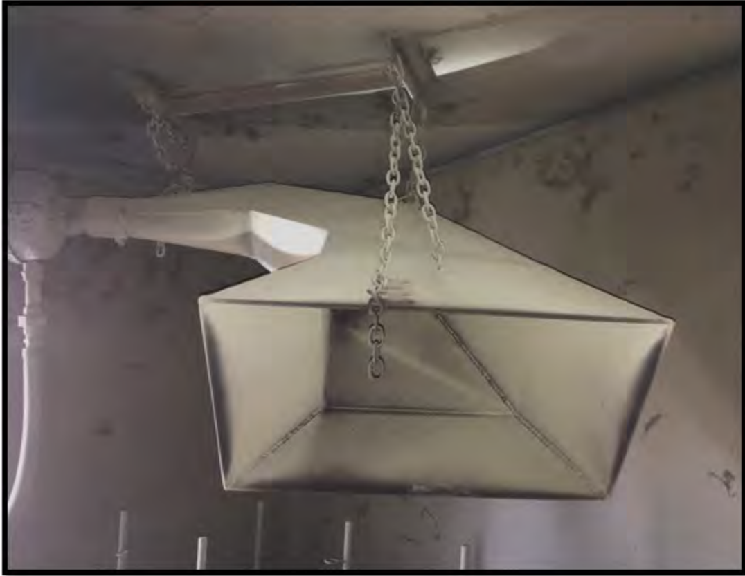
The bell is in good condition.
